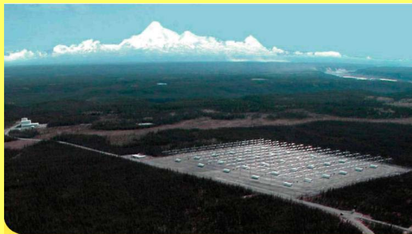
Fig. 25: HAARP location and construction.
